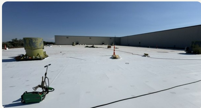
After: new heat-welded Duro-Last membrane.
